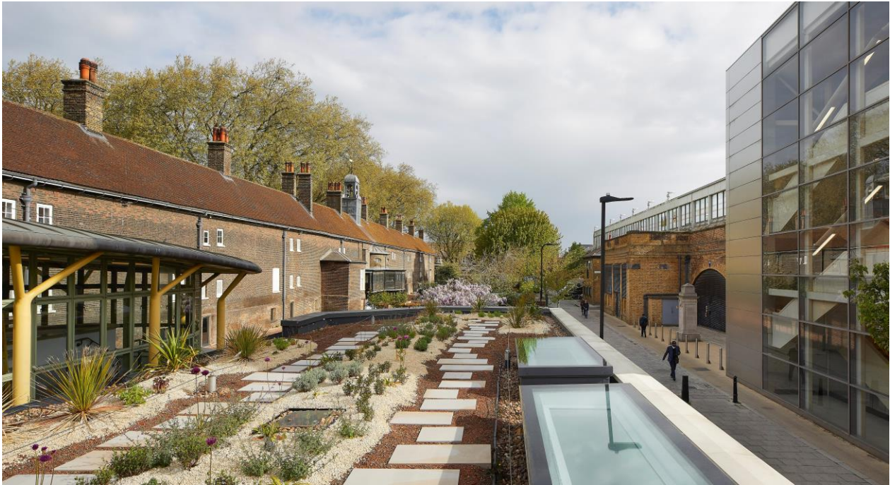
The green roof is a modern addition to the Gardens Through Time and can be admired both from the new reception space and from adjacent Hoxton Station, seen on the right. © Hufton & Crow
